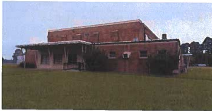
Figure 4 - View looking toward the Front of the Building - facing West.
