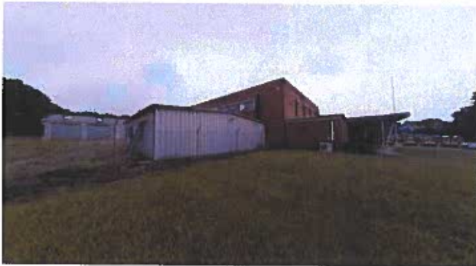
Figure 5 - View looking toward the South Facade of the Building - facing North.
