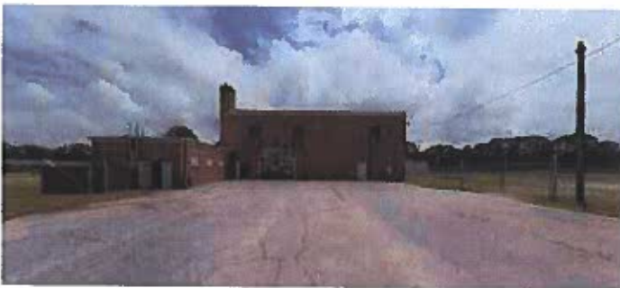
Figure 6 - View looking toward the Back of the Building - facing Southeast.
