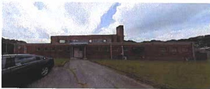
Figure 7 - View looking toward the side of the Building - facing Southwest.
