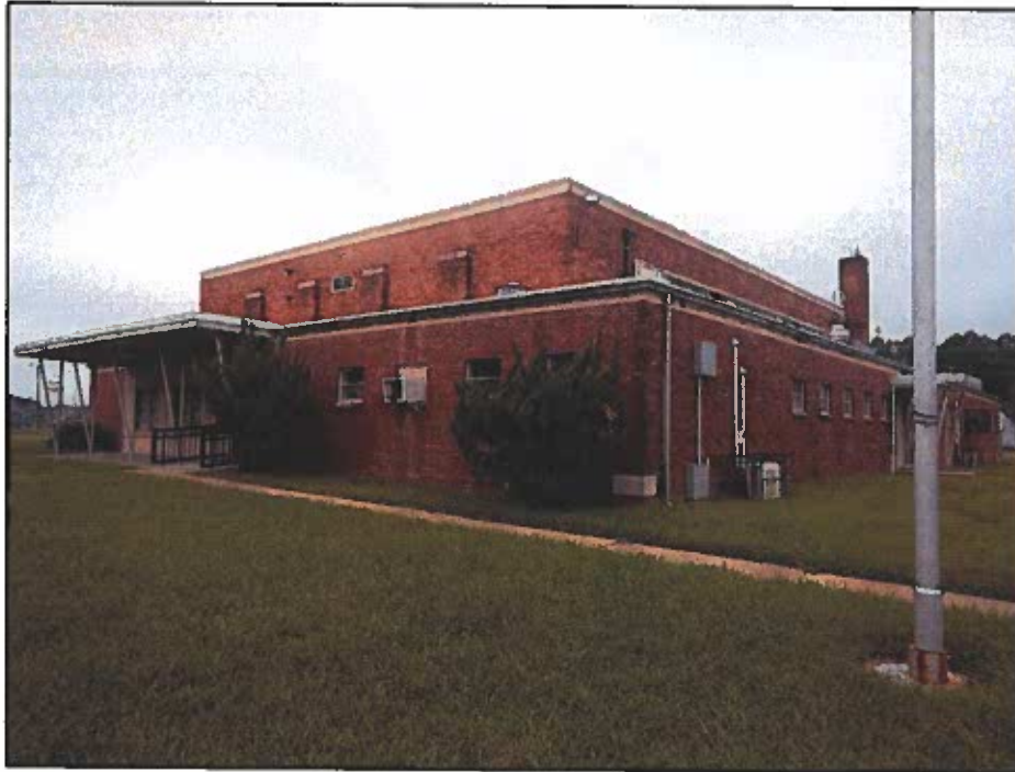
Photo 1: Front view of the Armory Building
