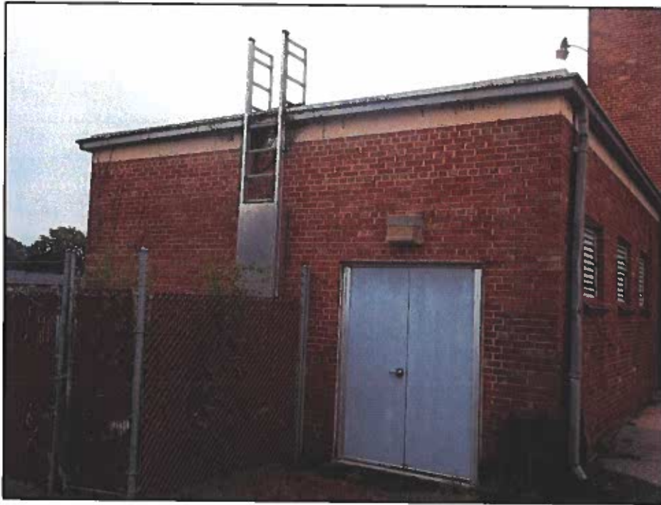
Photo 9: Exterior of the mechanical room space
