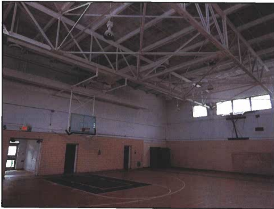
Photo 4: General Gymnasium Space
