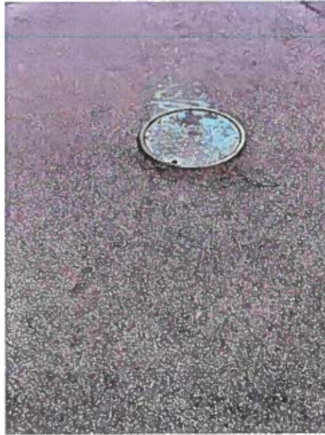
Manhole Protruding Above Pavement
