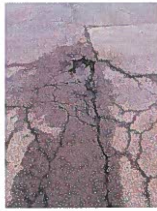
Patching, Alligator Cracking and Potholes in Laurel Street
