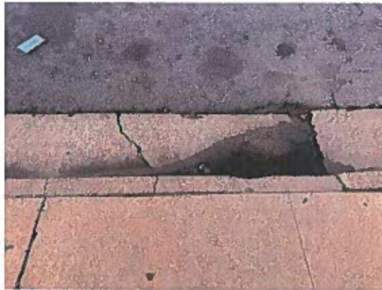
Cracked Curb and Gutter w/Differential Settlement
