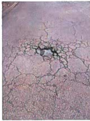
Patching, Alligator Cracking and Potholes in Laurel Street
