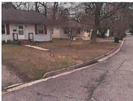
Low Spot, Differential Settlement
