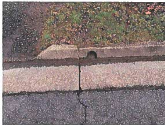
4" Roof Drain through Face of Curb
