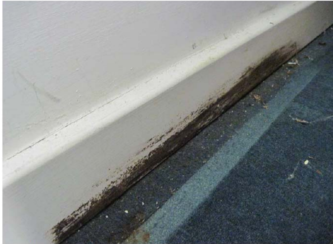
Photo 17: View of mold growth on wood wall base board, W wall under window.
