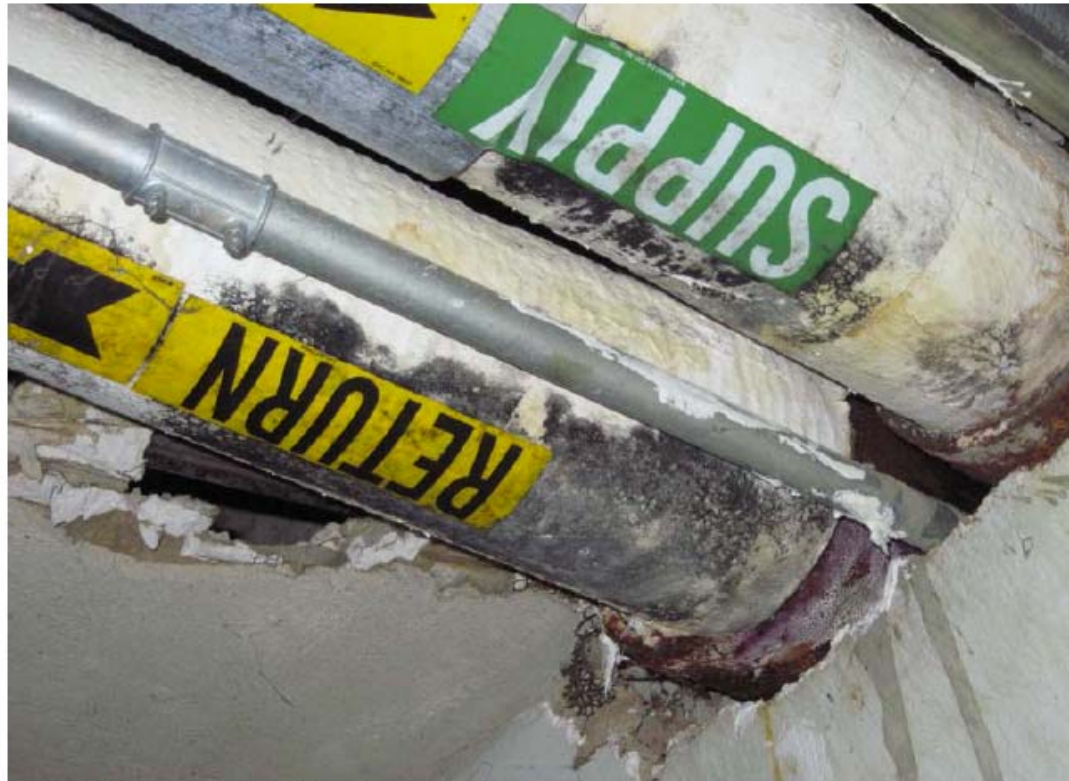
Photo 24: View of microbial growth on chiller lines.
