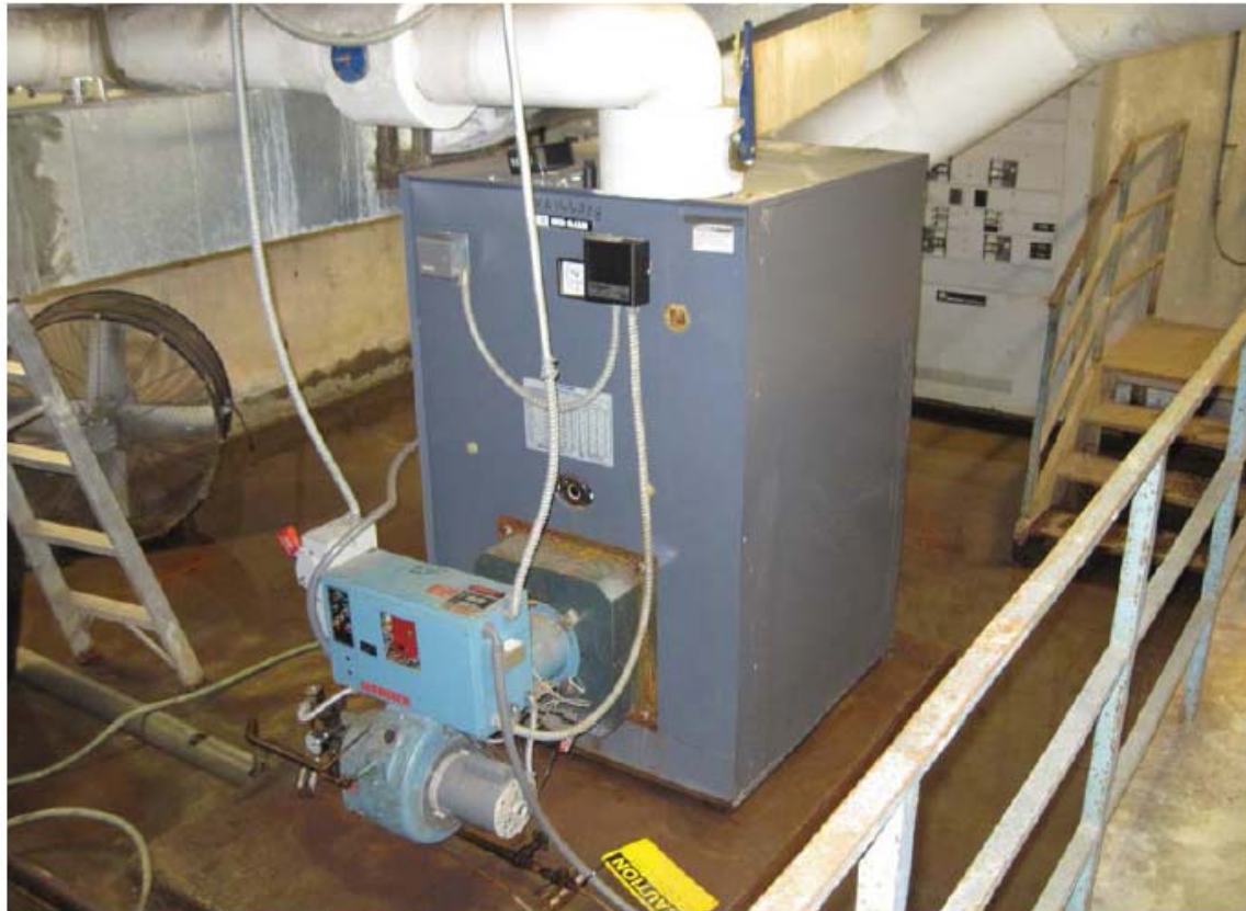
Photo 19: View of basemen boiler, water on floor.
