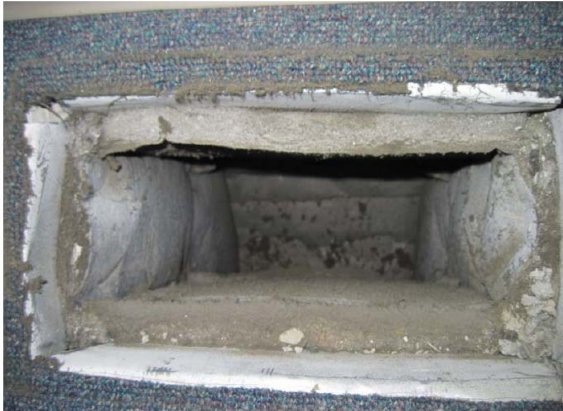
Photo 7: View of PH HVAC supply duct.
