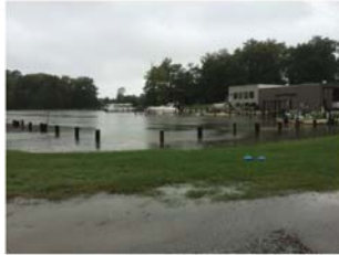
All the dry docks at the James City County Marina were underwater due to flooding last year. (Courtesy of Mark Gillespie)
