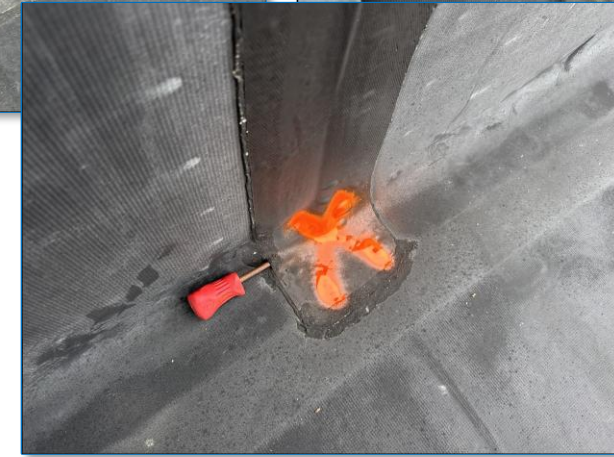
SEAM FAILURES AND AGE SHOWN DETERIORATION
