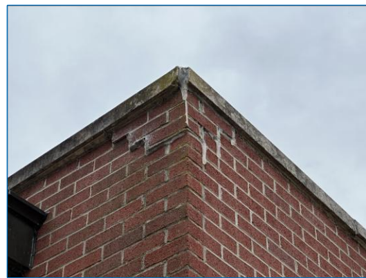
SEALANT FAILURES AND IMPROPER DETAILS HAVE LEAD TO WATER INTRUSION
