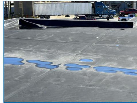
SEAM FAILURES AND SEALANT FAILURES AND IMPROPER DETAILS
