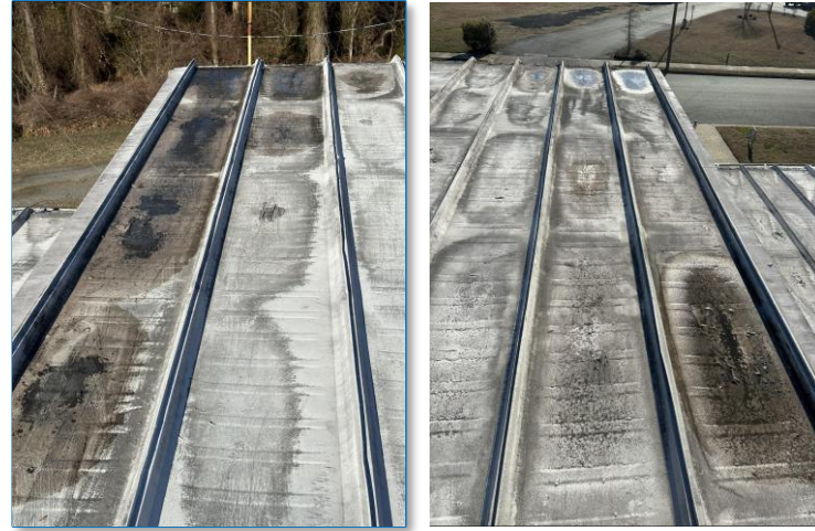
PONDING OCCURRING DUE TO DEPRESSION IN THE METAL PANELS
