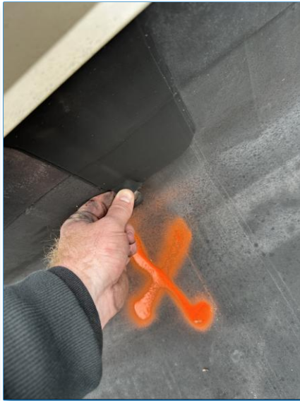
FAILURES AT THE SEAMS AND PREVIOUS REPAIRS
