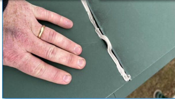
SEALANT HAS DETERIORATED. THE LOCATION OF POSSIBLE WATER INTRUSION AND LEAKS
