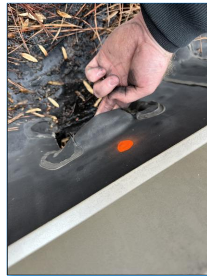
PONDING OCCURRING DUE TO THE SCUPPER DRAINS BEING TOO HIGH
