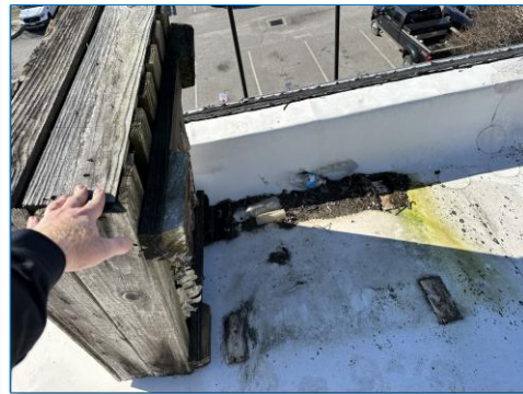
SLASHES / PUNCTURES THE LOCATION OF POSSIBLE WATER INTRUSION AND LEAKS
