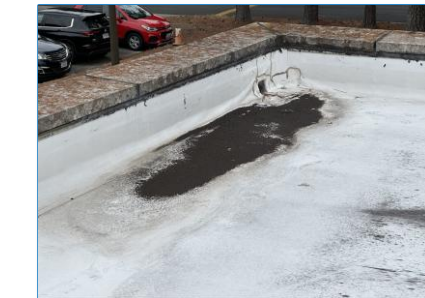
PONDING OCCURRING DUE TO THE SCUPPER DRAINS BEING TOO HIGH
