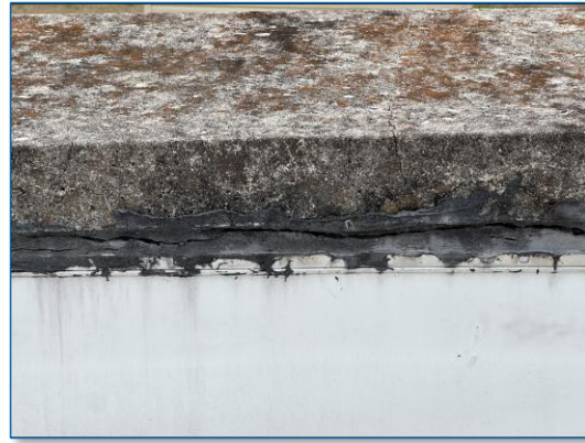
SEALANT FAILURES AND IMPROPER DETAILS HAVE LEAD TO WATER INTRUSION
