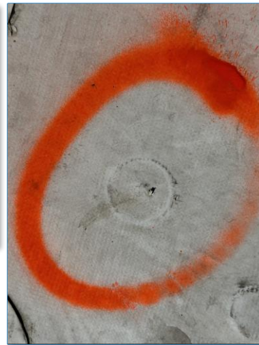
SLASHES / PUNCTURES THE LOCATION OF POSSIBLE WATER INTRUSION AND LEAKS
