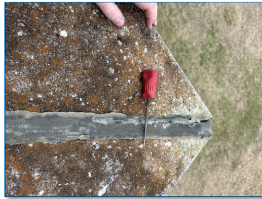
SEALANT FAILURES AND IMPROPER DETAILS HAVE LEAD TO WATER INTRUSION
