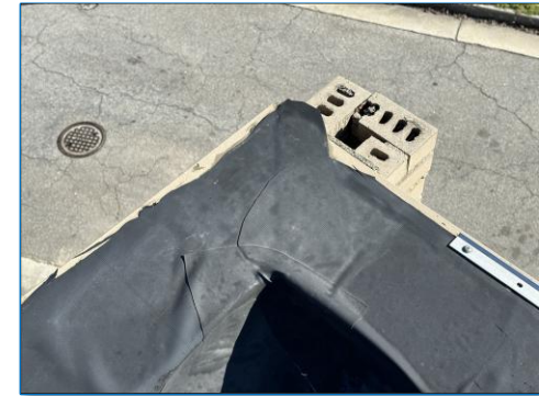
SEAM FAILURES AND SEALANT FAILURES AND IMPROPER DETAILS
