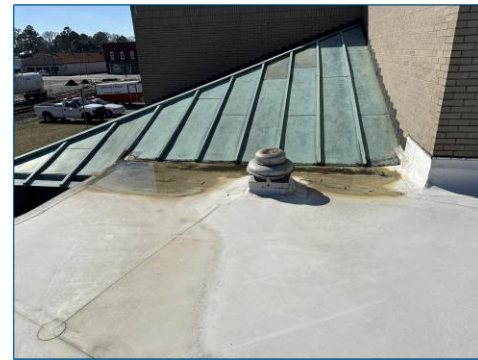
PONDING OCCURRING OVER DEPRESSED INSULATION
