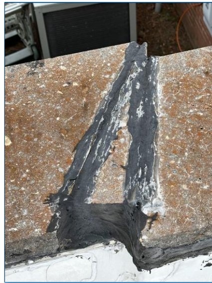
SEALANT FAILURES AND IMPROPER DETAILS HAVE LEAD TO WATER INTRUSION
