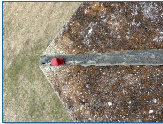
SEALANT FAILURES AND IMPROPER DETAILS HAVE LEAD TO WATER INTRUSION
