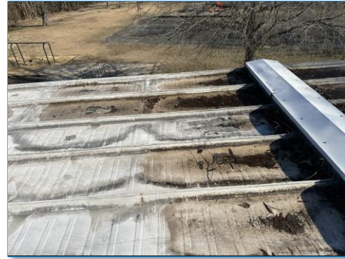
PONDING OCCURRING DUE TO DEPRESSION IN THE METAL PANELS
