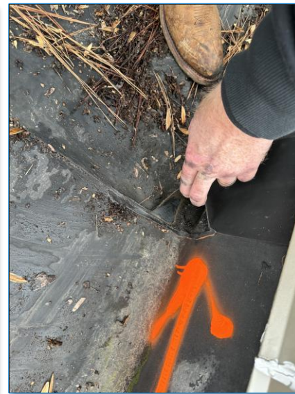
FAILURES AT THE SEAMS AND PREVIOUS REPAIRS
