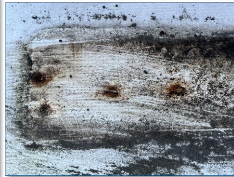
PONDING OCCURRING OVER DEPRESSED INSULATION
