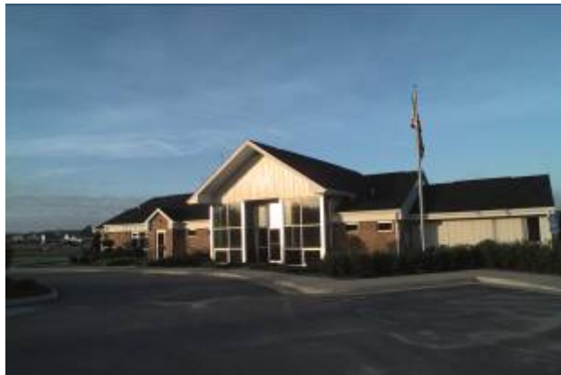
Franklin Municipal Airport
